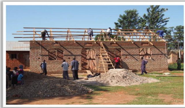
Classrooms being built by the German team
